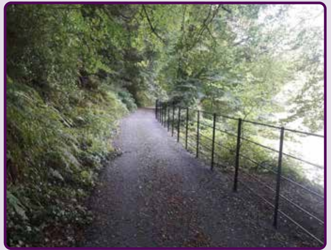
Woodstock walk loop – trail surface upgraded & new railing
