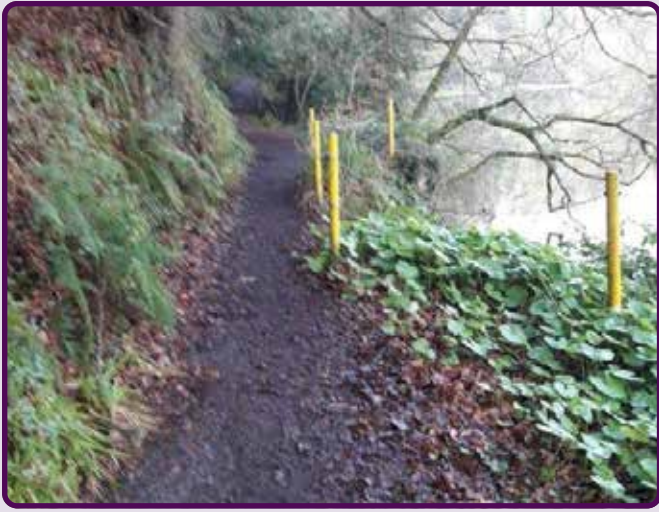
Woodstock walk loop – poor surface and chain link
