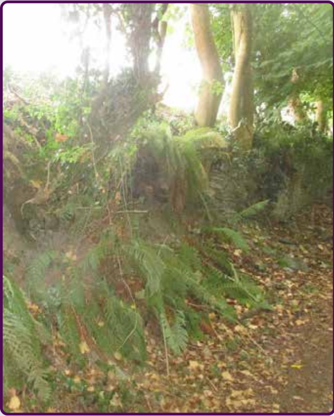
Ladies loop – collapsed wall
