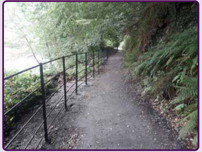
Woodstock walk loop – trail surface upgraded & new railing fence
