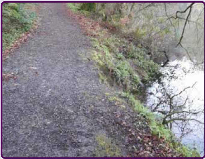
Woodstock walk loop – poor surface and dangerous edge
