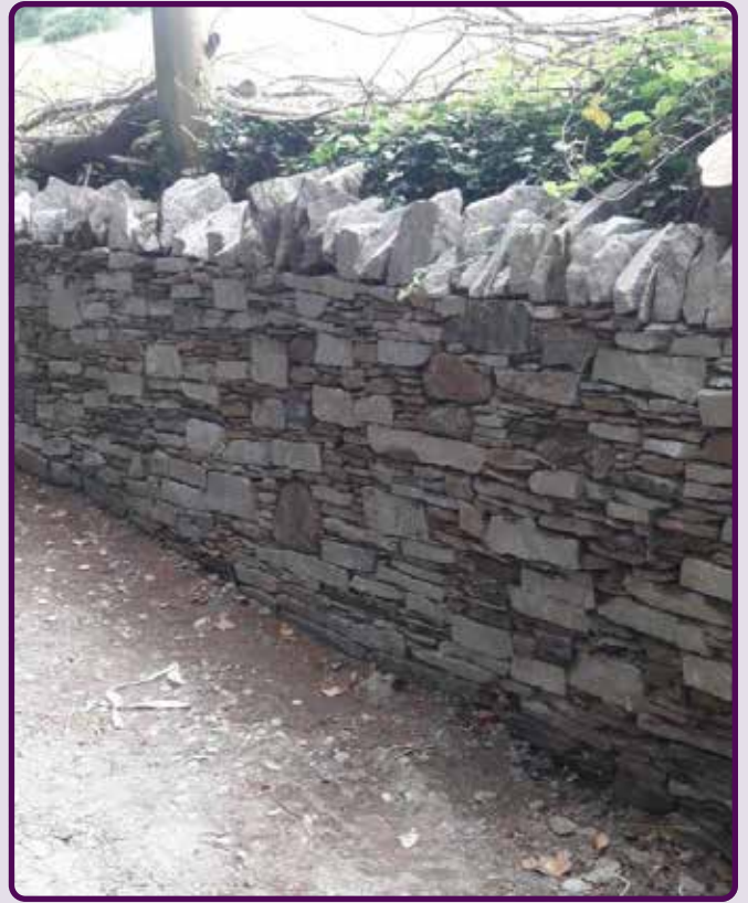
Ladies loop – wall repairs
