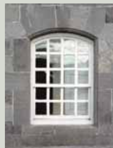
The substantial joinery seen here in a window of the 1720s had an aesthetic purpose as well as a practical one. The strong grid was thought to contribute to the character of the architecture
