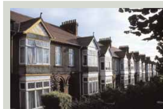
This terrace of thirteen houses was built in 1907. Almost all retain their original windows of stocky timber casements which contain decorative toplights
