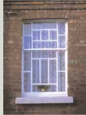
The top light of this decoratively designed metal window is a pivot, which swings about its horizontal axis (the top swings inwards and the bottom outwards)
