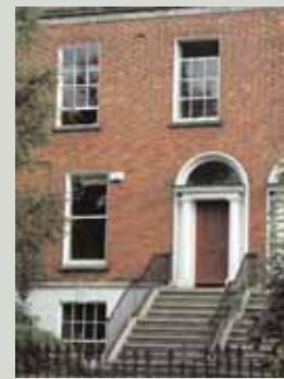
Fitting plate glass was a fashion statement. Using a hierarchy of plate glass for the main rooms and small-paned sashes for basement and bedroom floors became commonplace in the late nineteenth century
