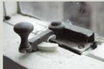
The meeting rails must line up accurately for quadrant fasteners to close properly, as was done when this window was repaired
