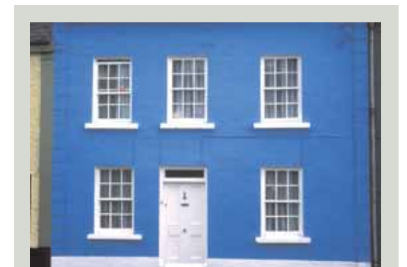
The original sash windows in this house seemed to be cared for - like the house generally
