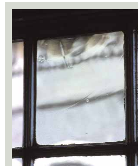
Crown glass was blown into a sphere and cut and spun by centrifugal force into a disc of very thin glass. Most panes have a characteristic curve and some are bowed or bellied. All have a soft polished appearance: some have a greenish tint like this one, while other panes can be quite purple
