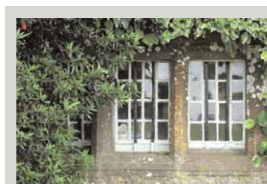
Lead-glazed fixed lights and casement windows of the seventeenth century are extremely rare in Ireland. Called 'quarry glazing', lead panels were still being made into the early eighteenth century, but were seen as inferior to timber-framed windows in every way
