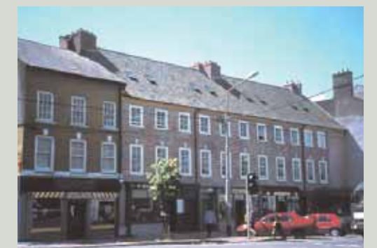
This restored terrace of early eighteenth-century houses retains the original appearance of the fully visible sash frames, which is quite different to the later house on the left
