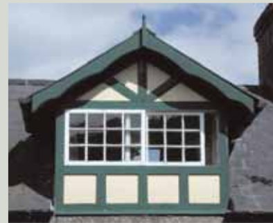
One side of a horizontal sliding window (sometimes called a Yorkshire sash) can be pushed open, while the other is fixed shut
