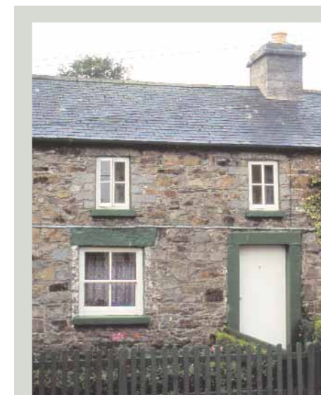
Timber casement windows were cheaper to make than sashes, and so were often the choice of those housing workers. Here they are used in the bedrooms, letting the main living room have the more prestigious sash window
