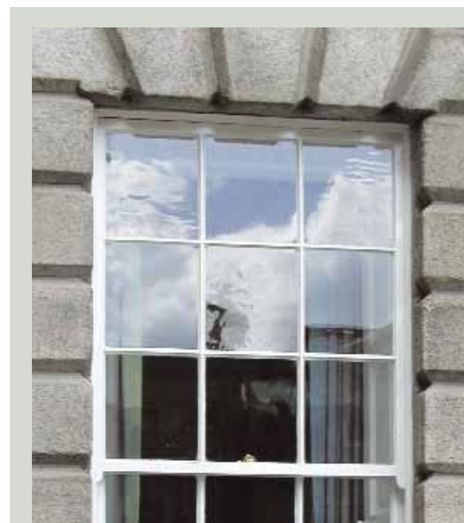
This sash was glazed with modern cylinder sheet glass. Each sheet of this or any other substitute for historic glass should be carefully examined before using it, as some, especially those sold for stained glass work, contain exaggerated imperfections and will look out of place
