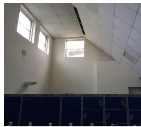
View of ceiling to Locker Room
