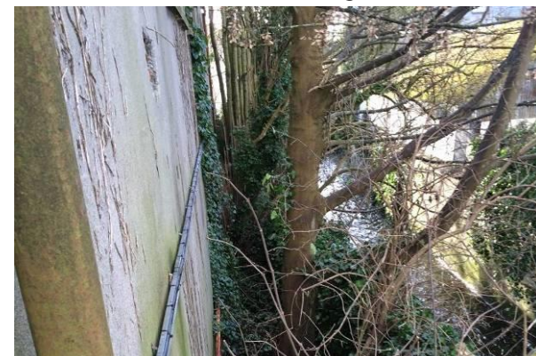
View west long walkway between Mayfair and Breaghagh River
