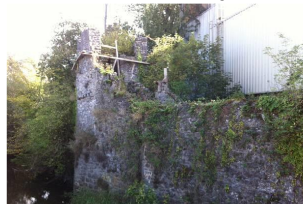
View east from Breaghagh Bridge to Evan's Turret
