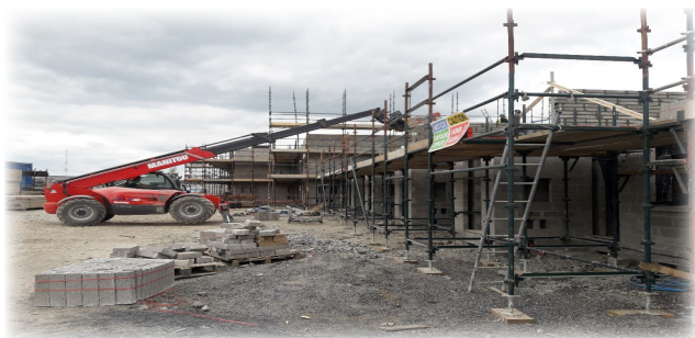
Works ongoing at Pennefeather Green, Hebron Road [Turnkey Project – 66 units]
