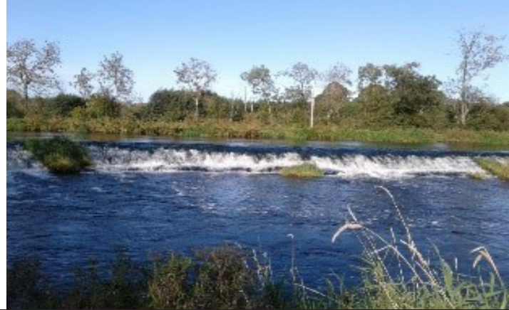
View of the weir on the River Barrow from Cois Bearbha
