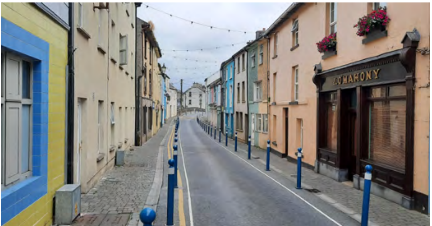
Mobility Management works at Bridge Street, Callan
