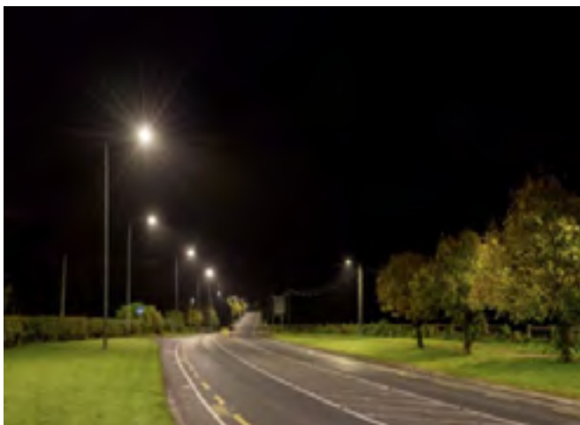
The Public Lighting Energy Efficiency Project will reduce energy use in public lighting by at least 70%.
