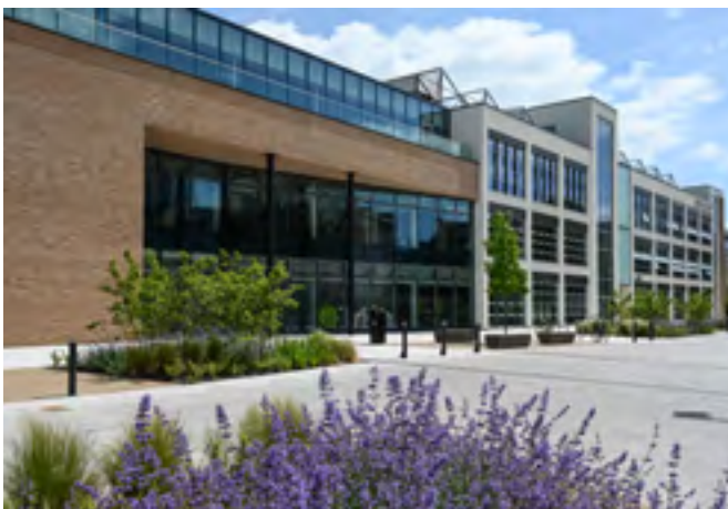
The Brewhouse, Abbey Quarter, has achieved LEED Gold rating, the highest rating of green building design
