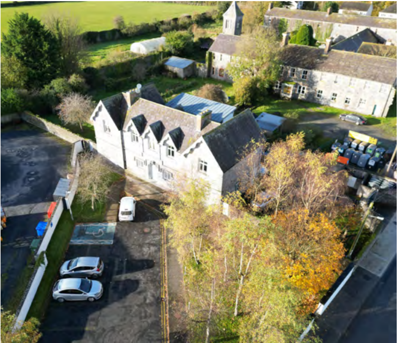
Many historic buildings such as the Callan Area Office, built in the 1840's, are not very energy efficient. So Kilkenny County Council has commissioned energy audits to identify measures which can be taken to reduce heat loss, whilst respecting the integrity of the building.
