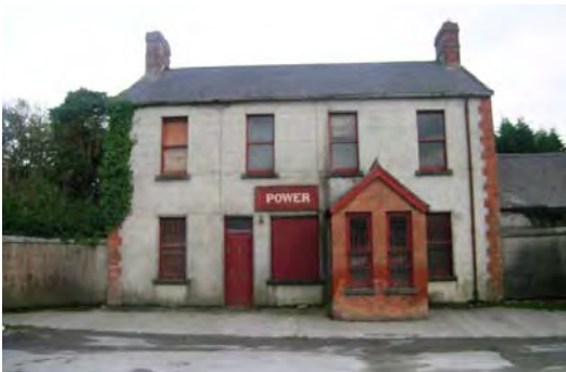
Main façade of pub
