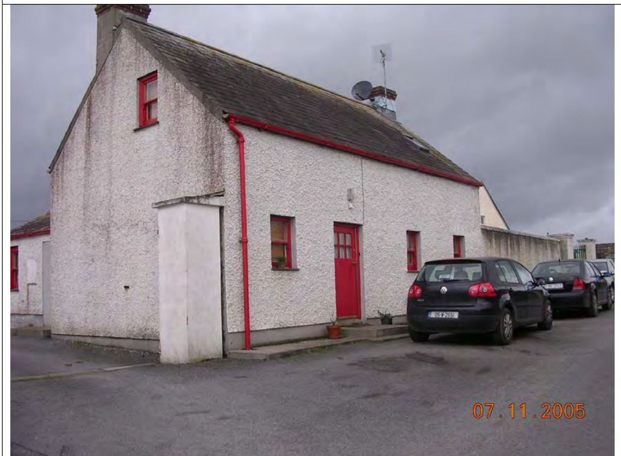
Plate 18. Looking northwest at AH4
