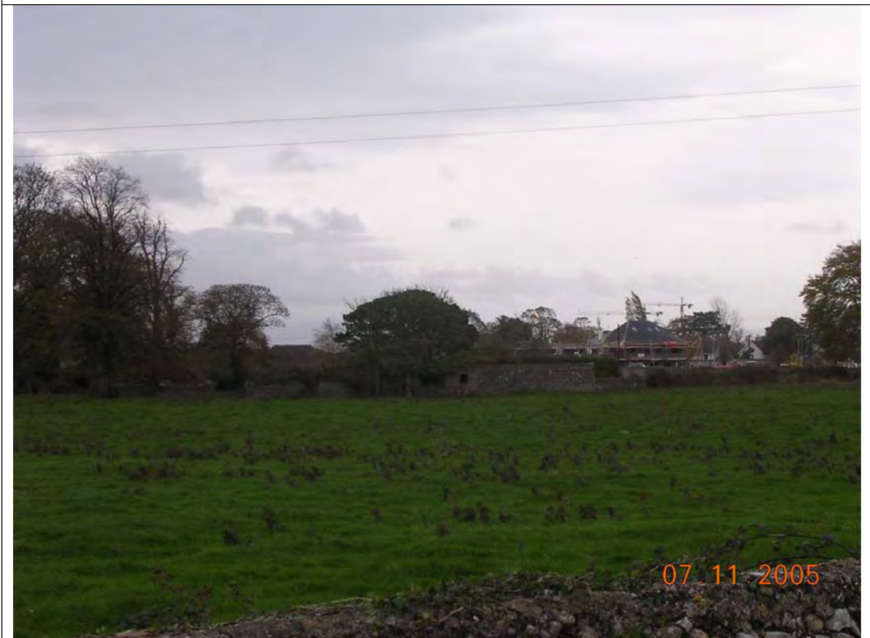
Plate 24. Looking east at AH7 (rear)
