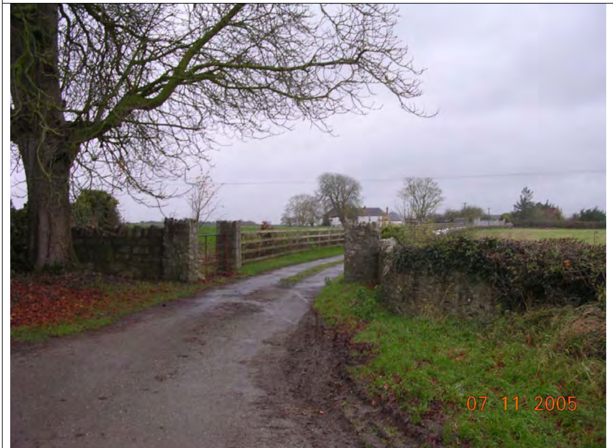
Plate 28. Looking west towards AH11.
