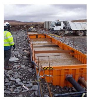
Figure 7-11 Settlement Tanks [Source SEPA Engineering in the Water Environment Good Practice Guide Temporary Construction Methods]
