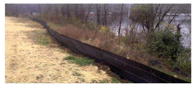
Figure 7-13 Silt Fence Installed alongside Riverbank [Source Thrace Synthetic]
