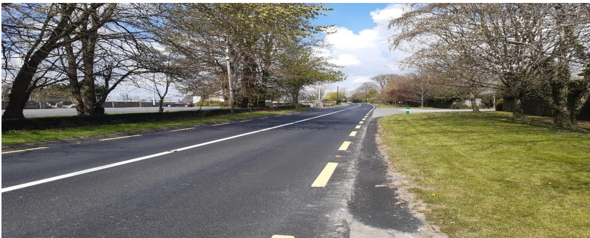
N78 Baun to Hennebrys Cross- Finished Pavement at Dunmore
