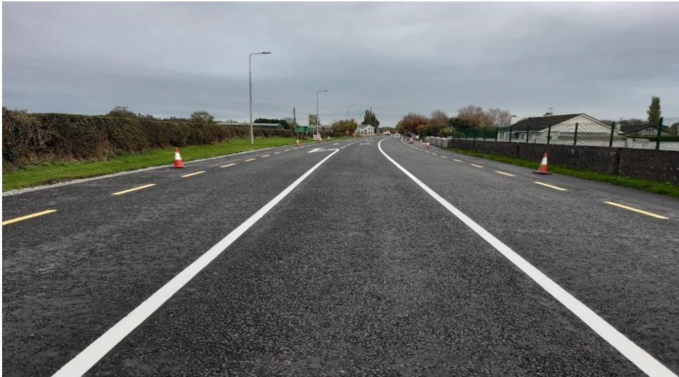
N77 Oldtown to Ballyragget – Finished Pavement
