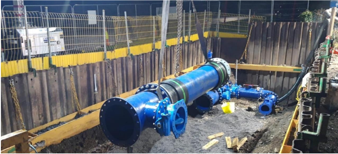
PRV installation at Radestown WTP
