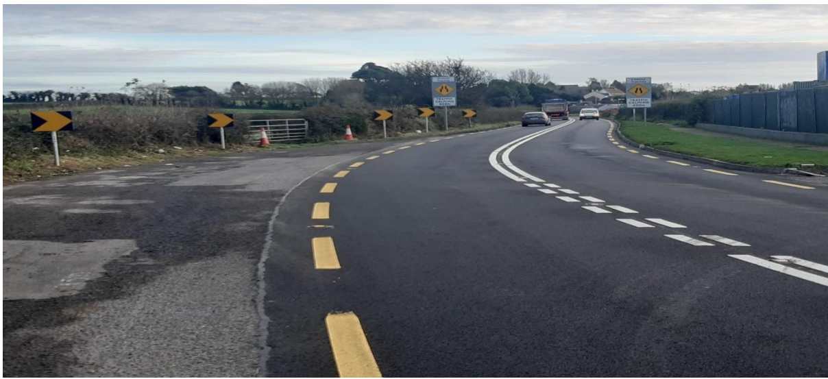
N24 West of Mooncoin. Renewed pavement, markings and signage.
