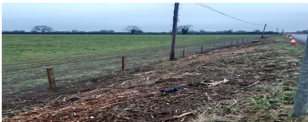
Typical Fencing Retrofit completed works on the N76
