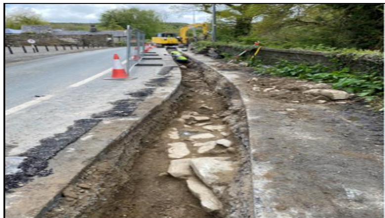
Construction of new HDPE water-main at Jerpoint Abbey
