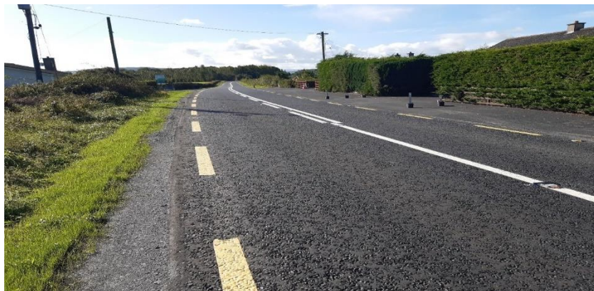
N76 Riversfield to Ahanure North – Finished Pavement
