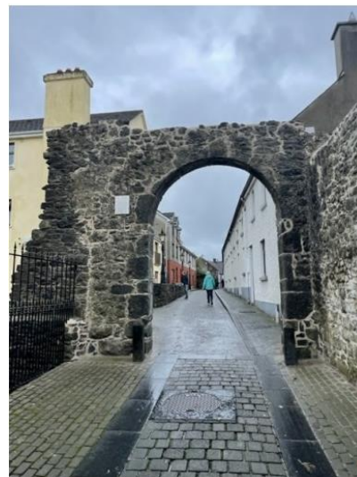
Black Friars Arch after repair and conservation works completed
