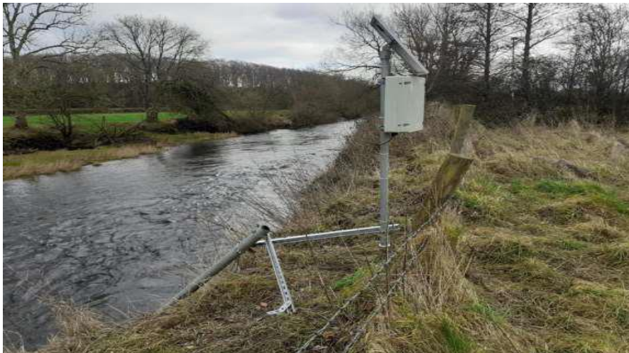
Water Quality Monitoring Station
