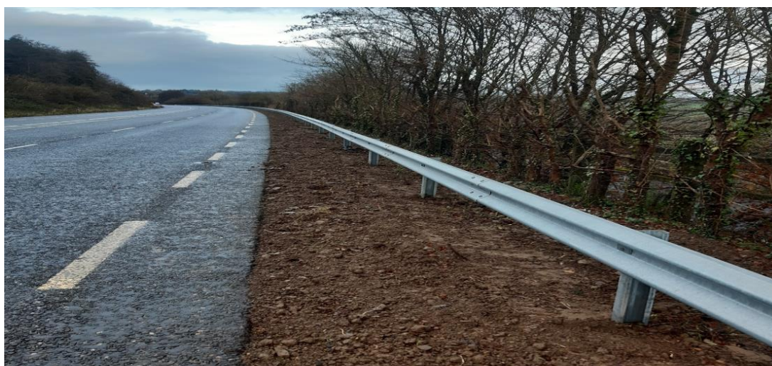
New section of VRS on the R723 (Former N25)
