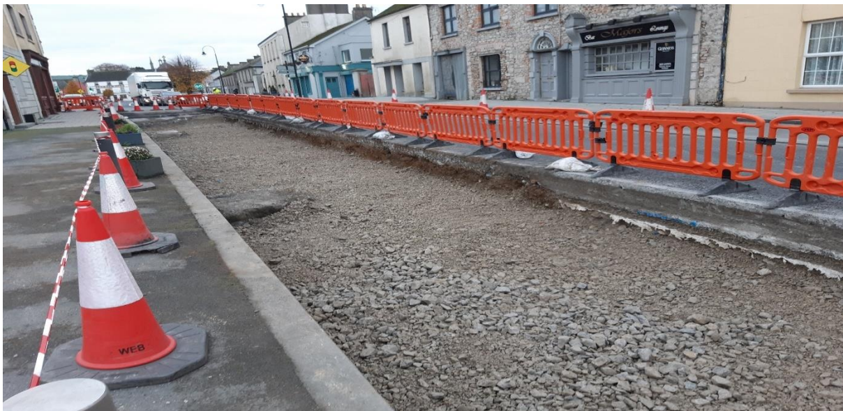
N77 Ballyragget- Works in progress on the reconstruction of failed pavement
