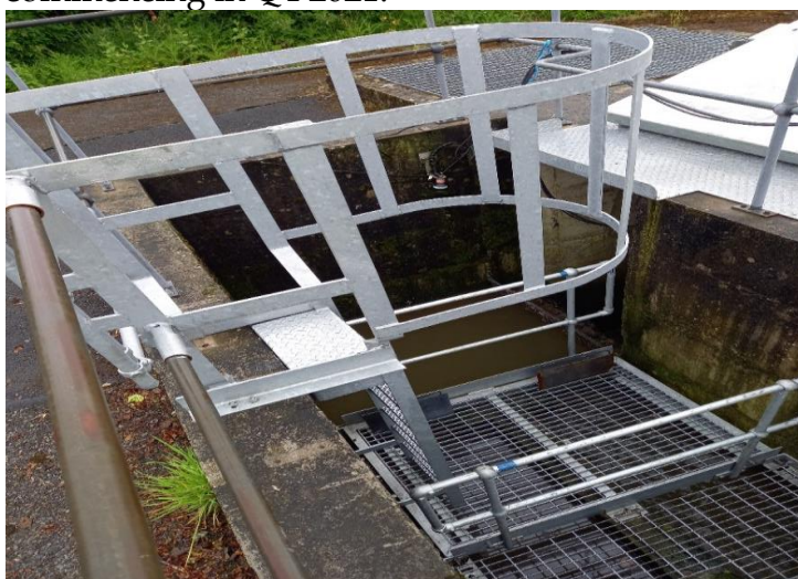
New Access Platform with Handrail support at Paulstown WWTP
