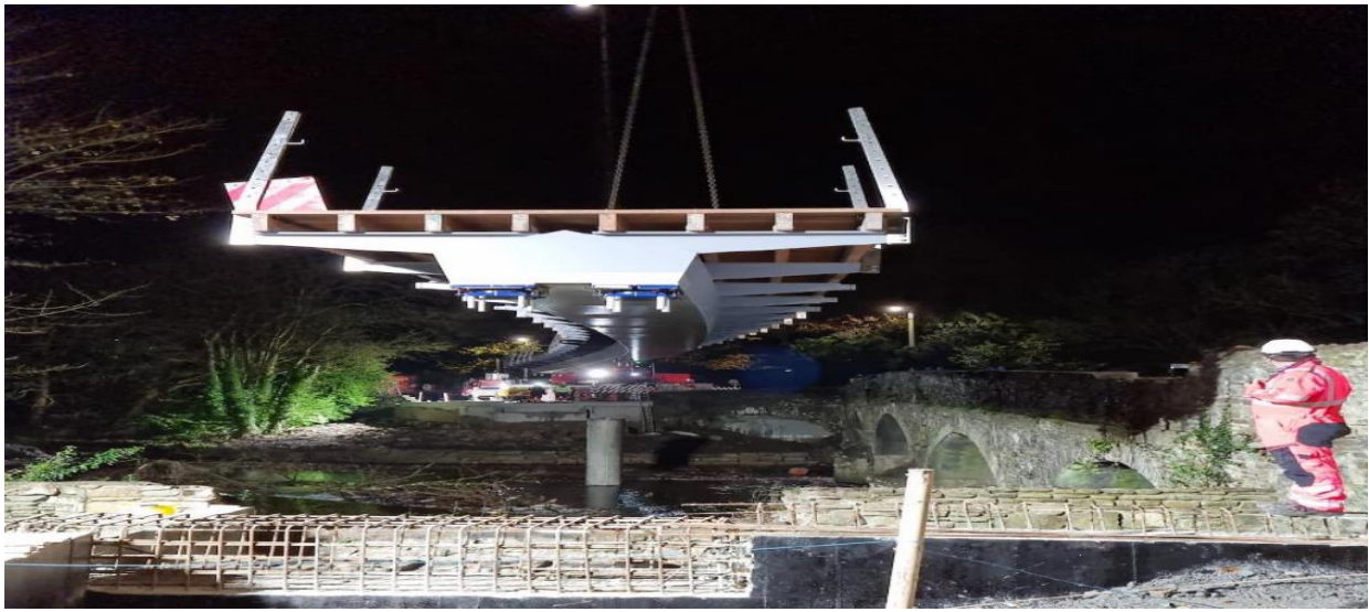
Bridge Lift in Progress around midnight on night of 23 rd November
