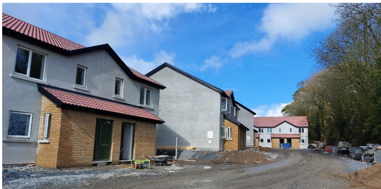
12 houses at The Crescent, Belmont, Ferrybank under Construction
