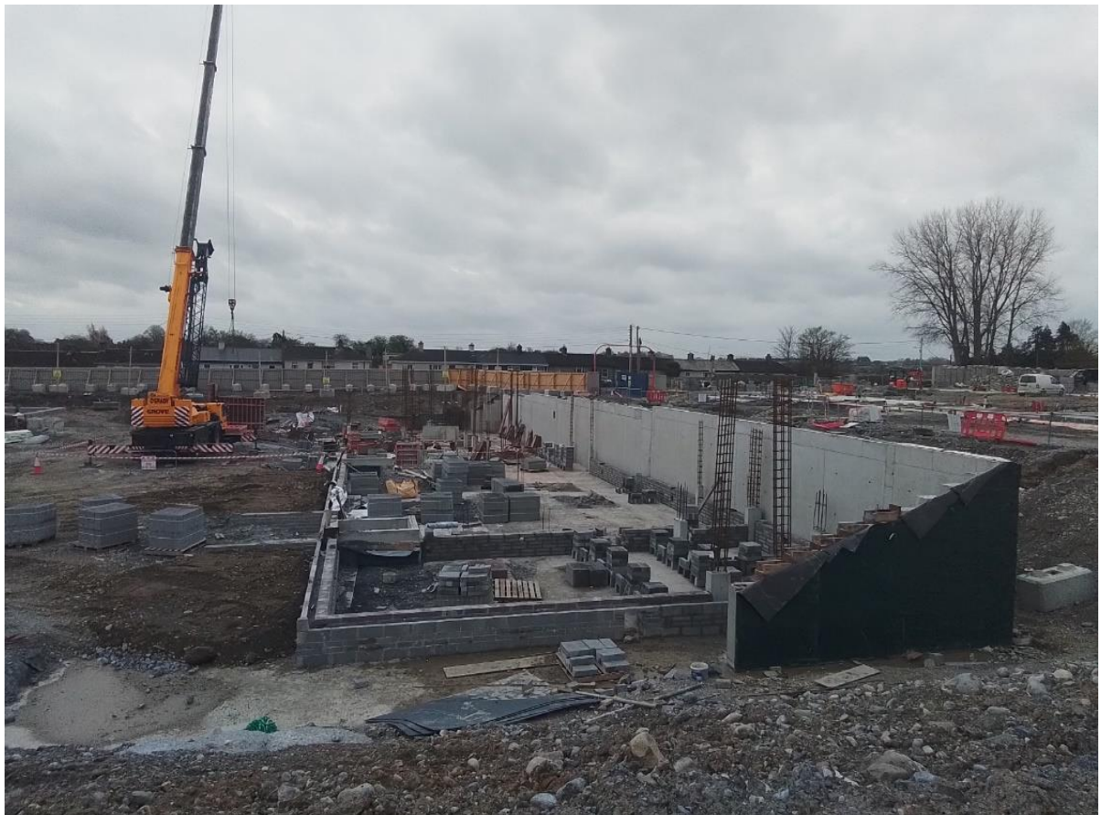
Construction at Crokers Hill, Kennyswell Road
