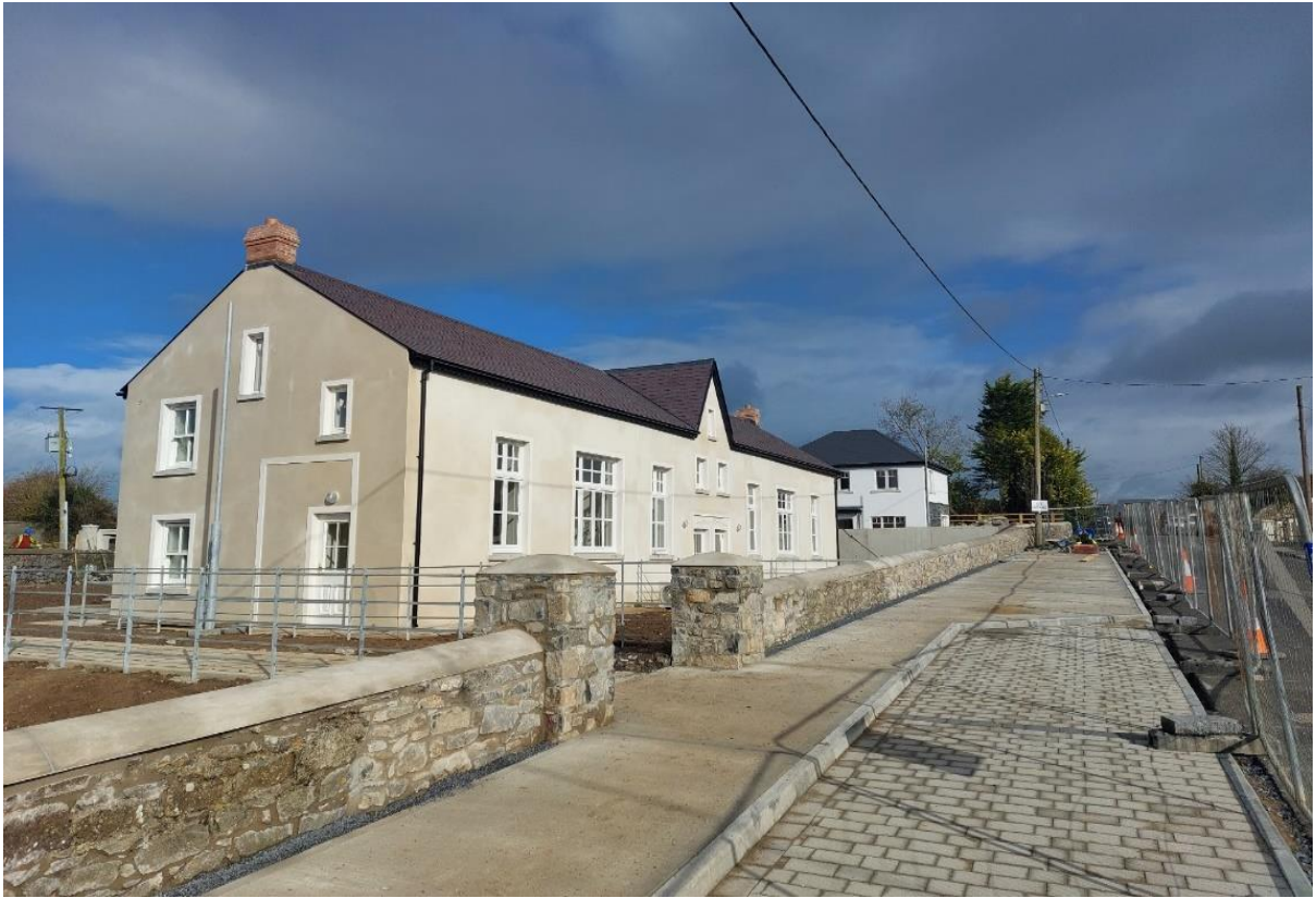
9 units at Old Creamery Kilmacow nearing completion
